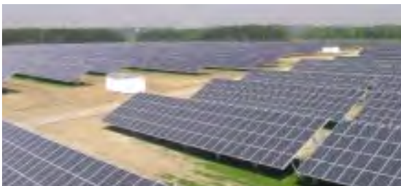
Fig. 2: How many kWp of PV power have been installed here? The power extrapolated from the data sheets, the manufacturer's measurements on individual modules or random samples by certified measurement laboratories always give different results. The "Performance" project will help to establish clear rules for the evaluation of large PV systems.
