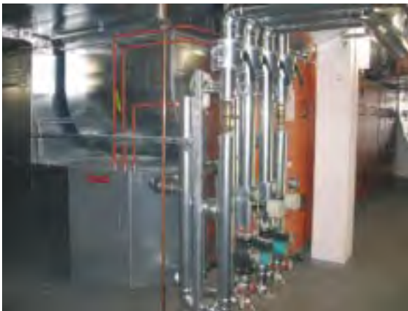
Fig. 1: Liqueorsorp project: Completely installed system in the Freiburg University Clinic. The photo shows the compact, orange-red housing of the air-conditioning equipment. In the foreground, the heating circuits for heating the brine in the regenerator (summer operation) and for heating the supply air (winter operation) can be seen.
