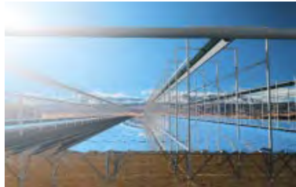
Fig. 1: Photorealistic simulation of a linear Fresnel collector array.
